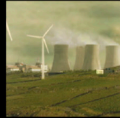
Nuclear Power Plant
